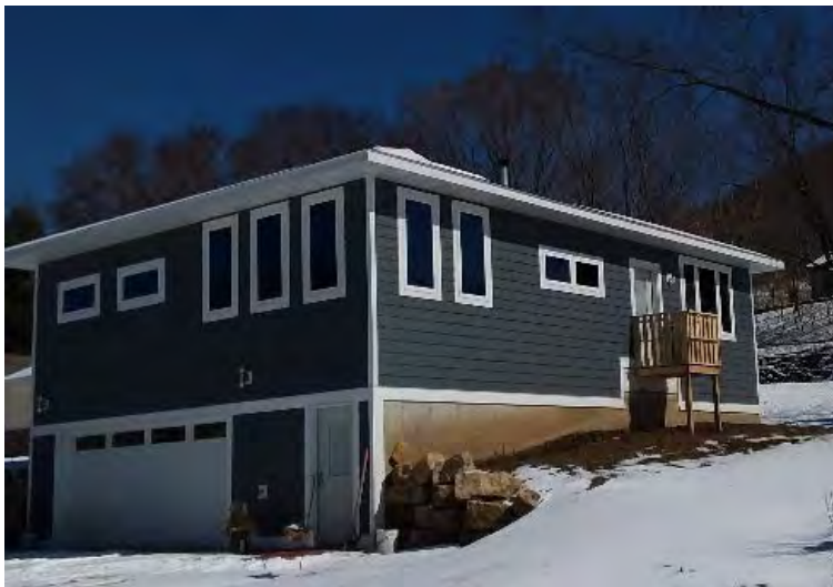
Figure 12. The single home with significant ductwork outside conditioned space.
