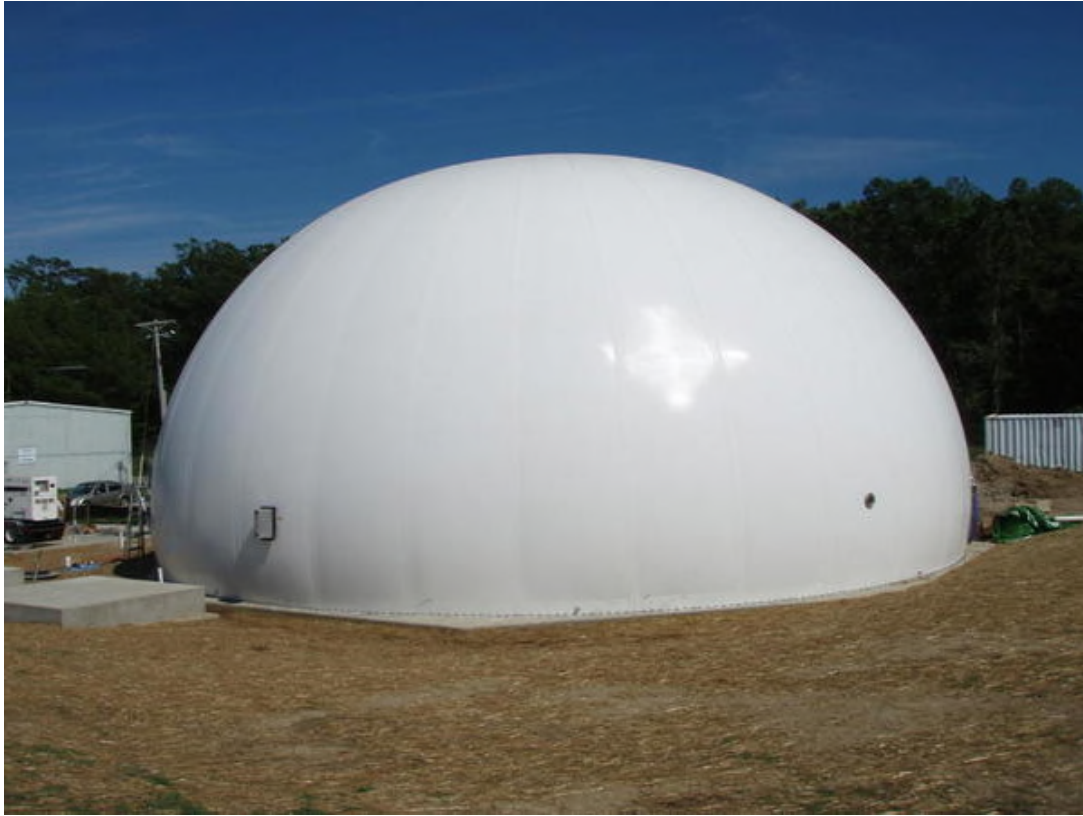
Figure 3-2. External Partial Dome on Concrete Slab
