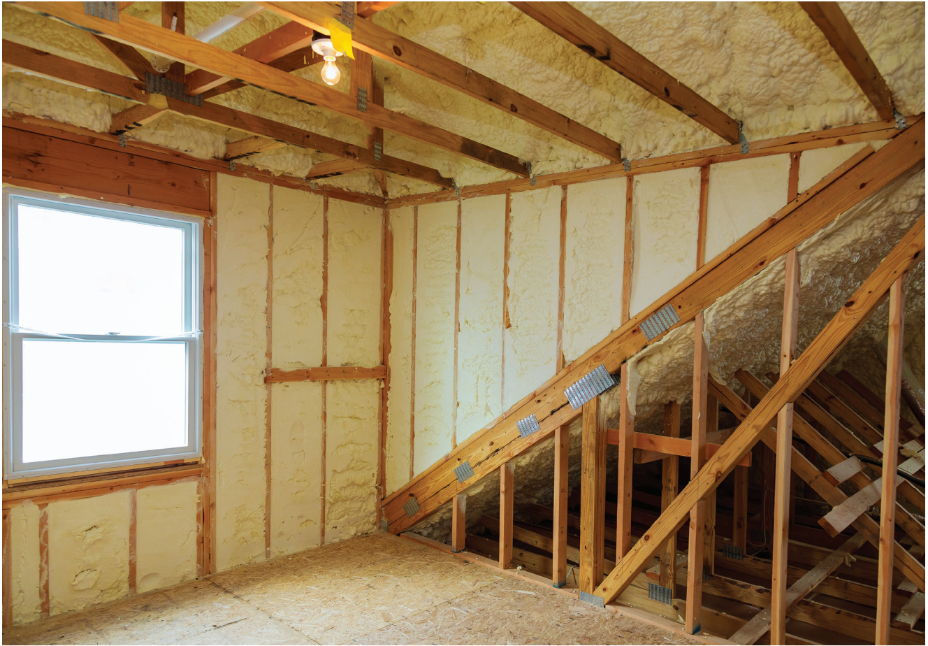
Spray foam installation
