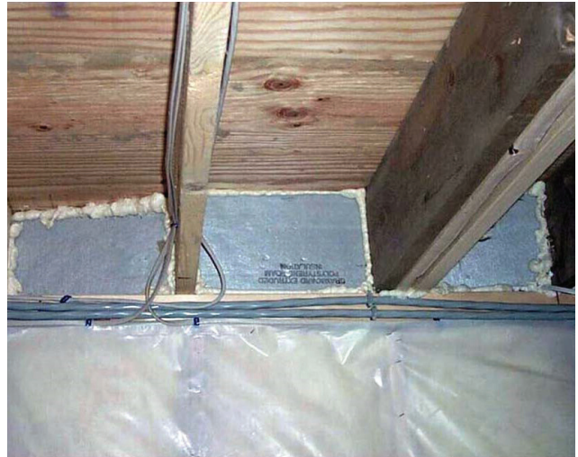
Rim join sealed to sill
