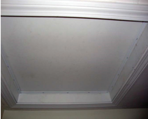
Attic hatch weatherstripped
