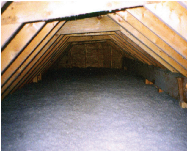
Loose-fill attic insulation evenly installed
