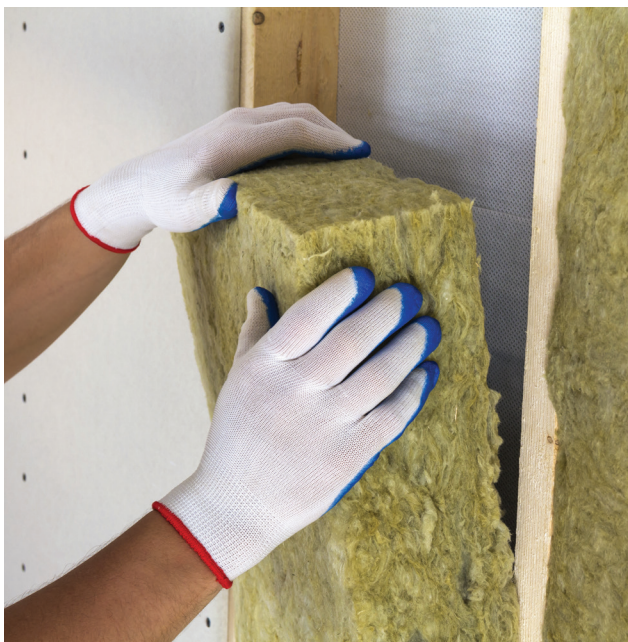
Insulate wall framing
