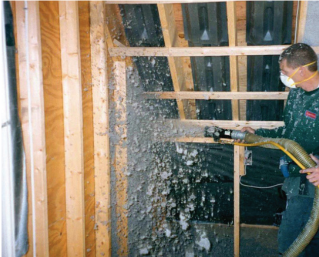
Roof line venting chute
