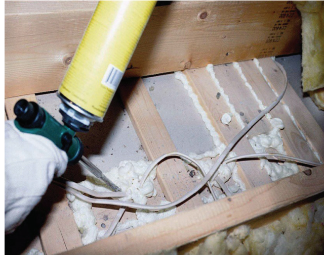
Top plates sealed with one-part foam
