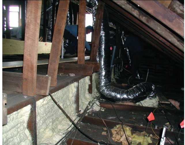
Ceiling height transition wall sealed with two-part foam
