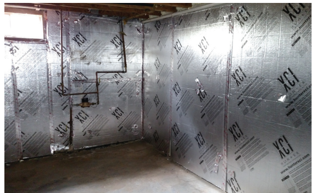
Basement and crawlspace insulation interior wall treatment
