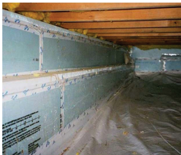
Crawlspace ground cover
