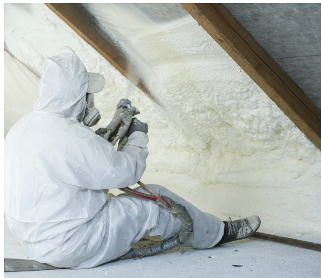
Spray foam installation in attic
