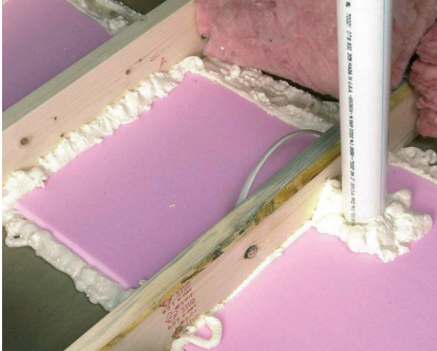
Dropped soffit sealed with XPS and one-part foam
