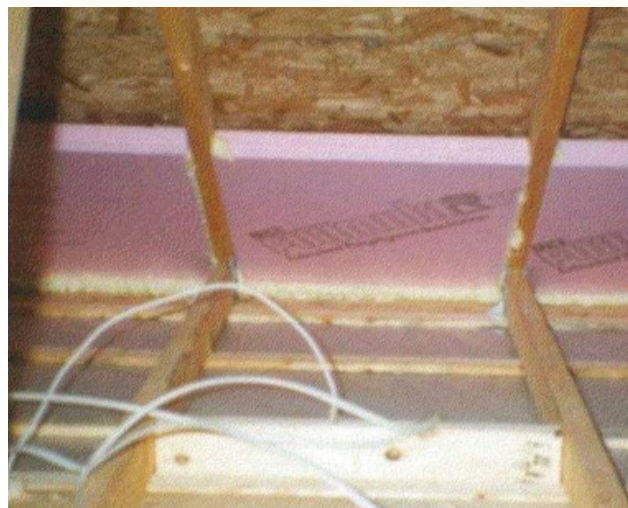
Insulation wind wash baffle
