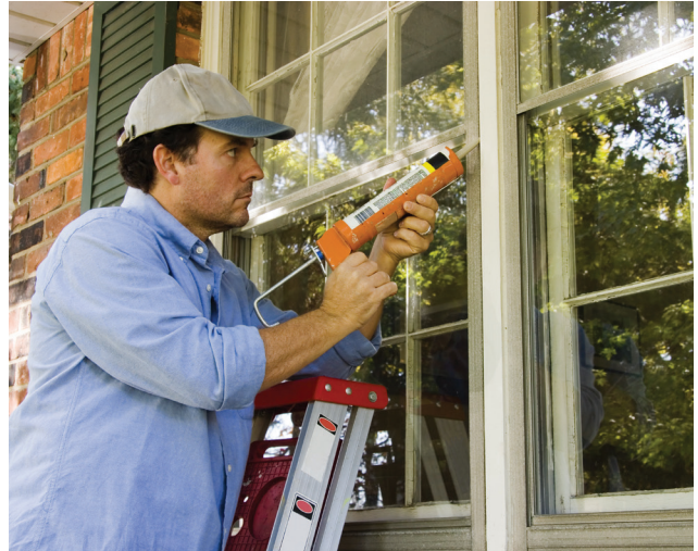
Applying caulk around window frame
