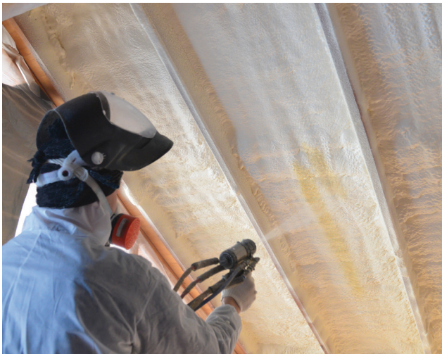
Spray foam installation
