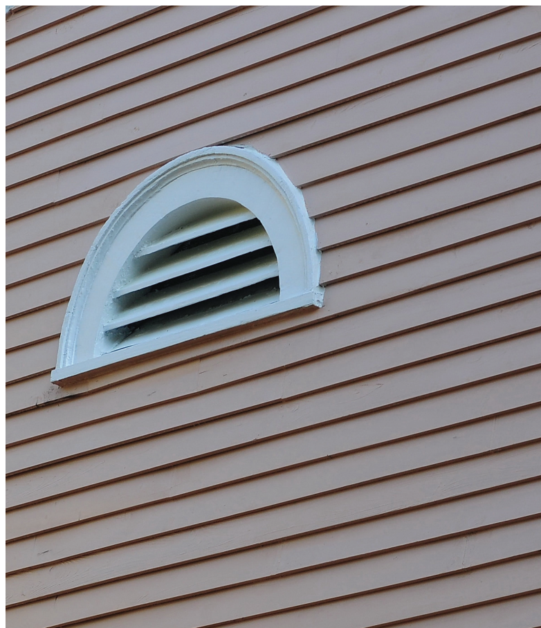
Attic eaves and venting
