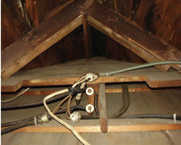
Knob and tube wiring
