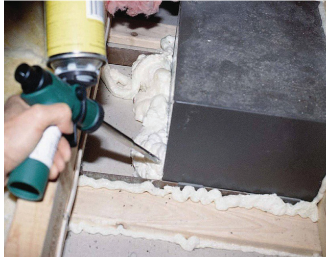
Bath fan sealed with one-part foam
