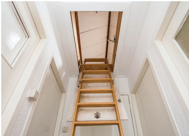
Attic hatch access
