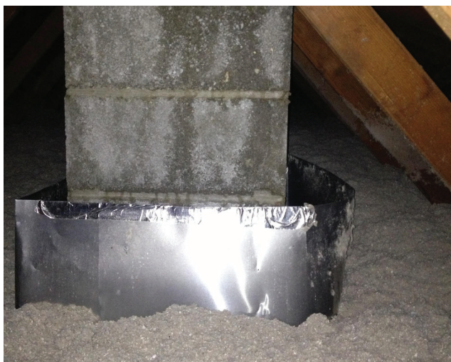
Flashed chimney with 3-inch spacing
