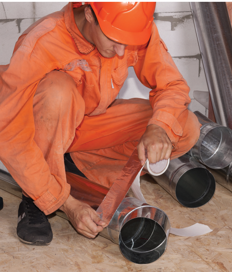
Sealing ducts
