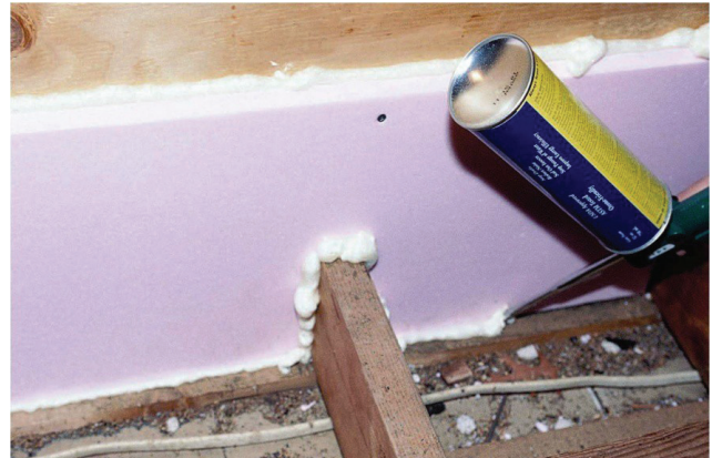
Knee wall transition sealed with XPS and one-part foam
