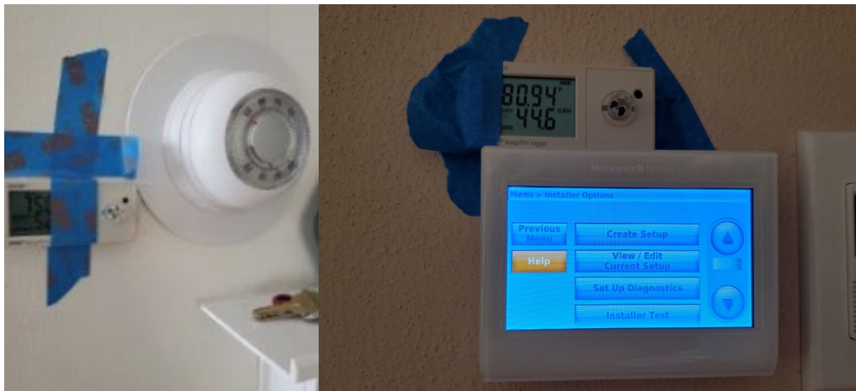
Figure 1: Temperature/RH HOBO loggers next to main floor thermostats.
