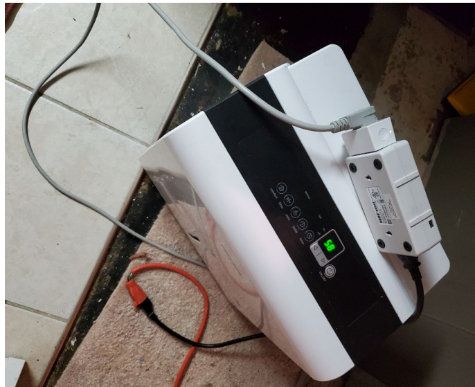
Figure 2: Plug load logger setup with dehumidifier and Wemo smart plug (site 6)
